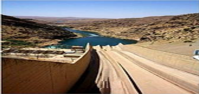
Figure 3. Spillway of Darbandikhan dam
